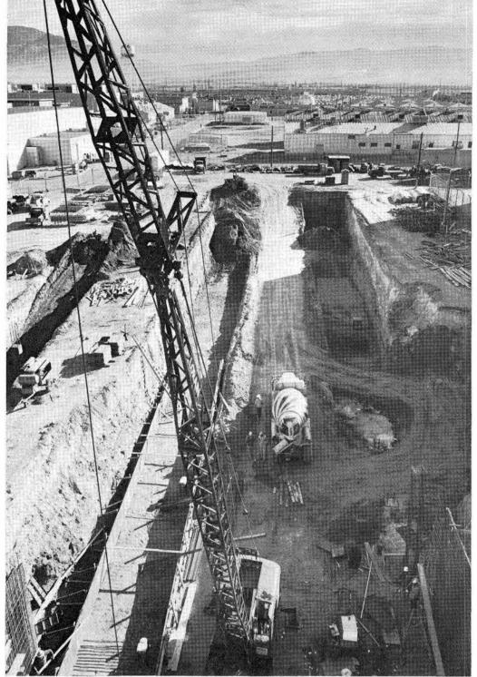
BLDG. 807 CONSTRUCTION currently in progress includes laying the foundation and basement concrete and construction of a utilities service tunnel. Photo was taken from the roof of Bldg. 806 which the new three-story laboratory building will adjoin. Scheduled completion date for Bldg. 807 is December 1965. C. R. Morrisett is the Plant Engineering Department project engineer.
